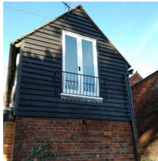
Use of brick on the ground level and timber on upper level, Goudhurst
