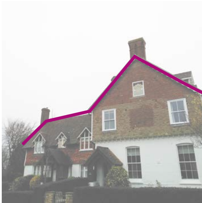
Three storey building on Rogers Rough Road, Kildown
