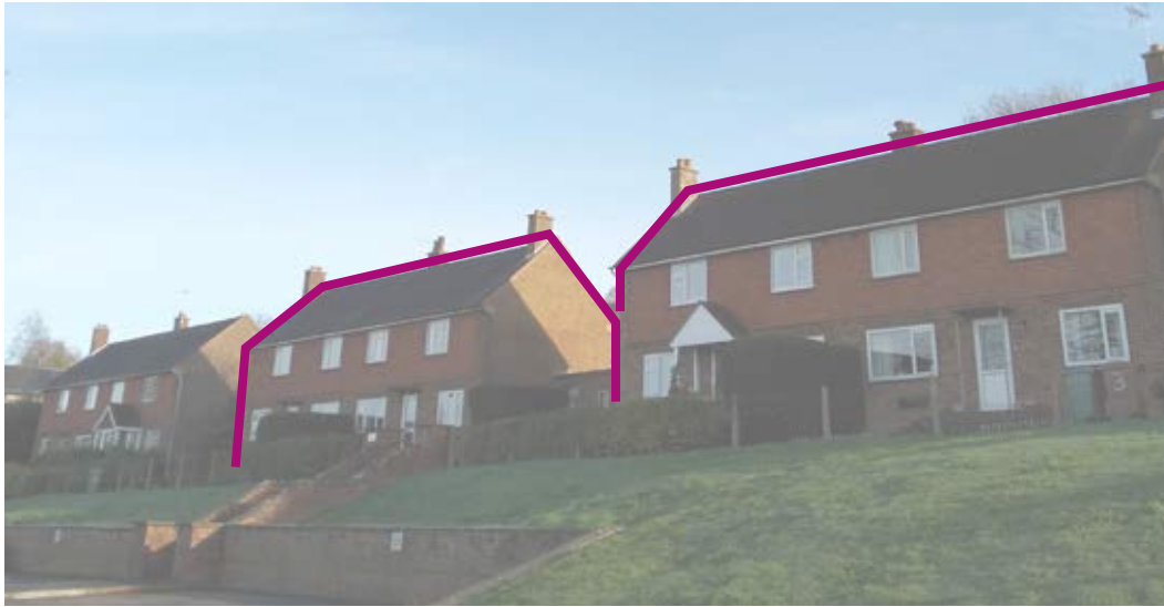
Two storey building on North Road, Goudhurst
